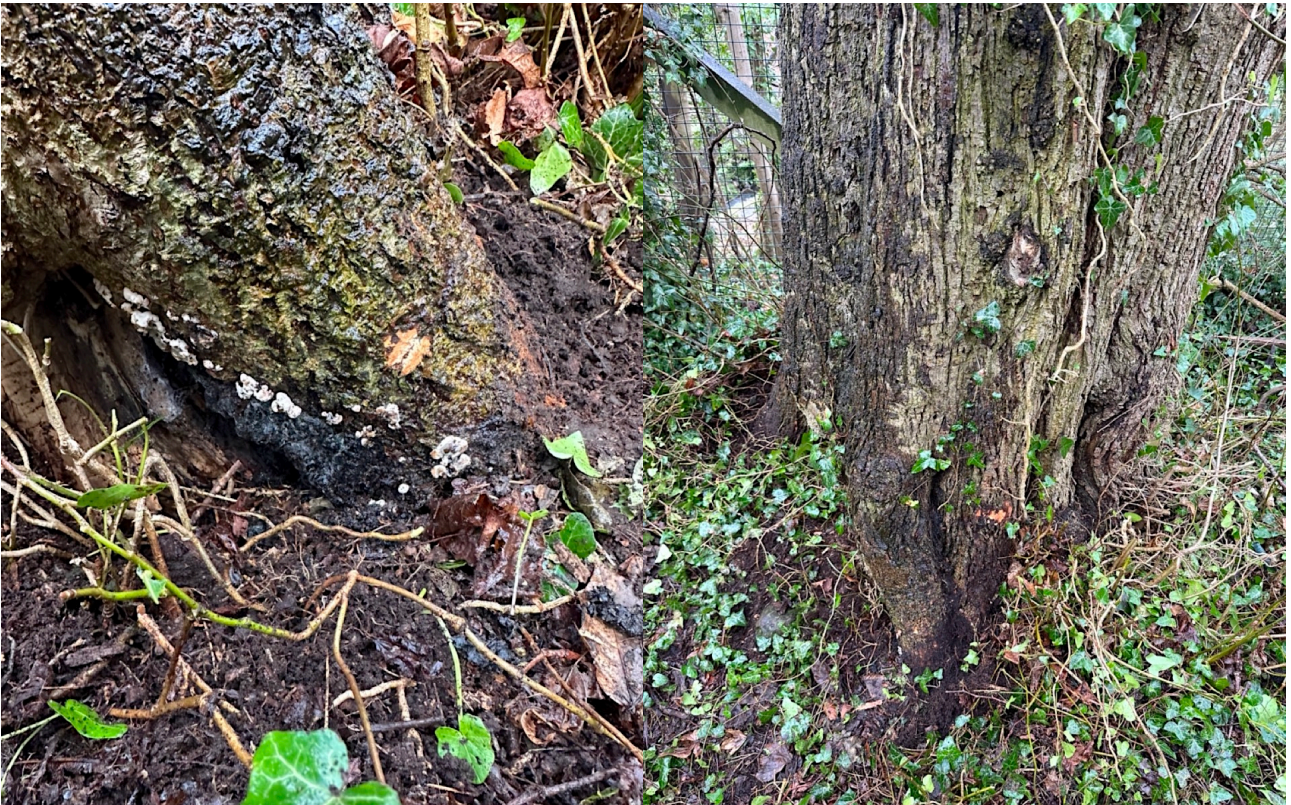
Photo 3: Lime (553). Buttress with Kretzschmaria deusta .
